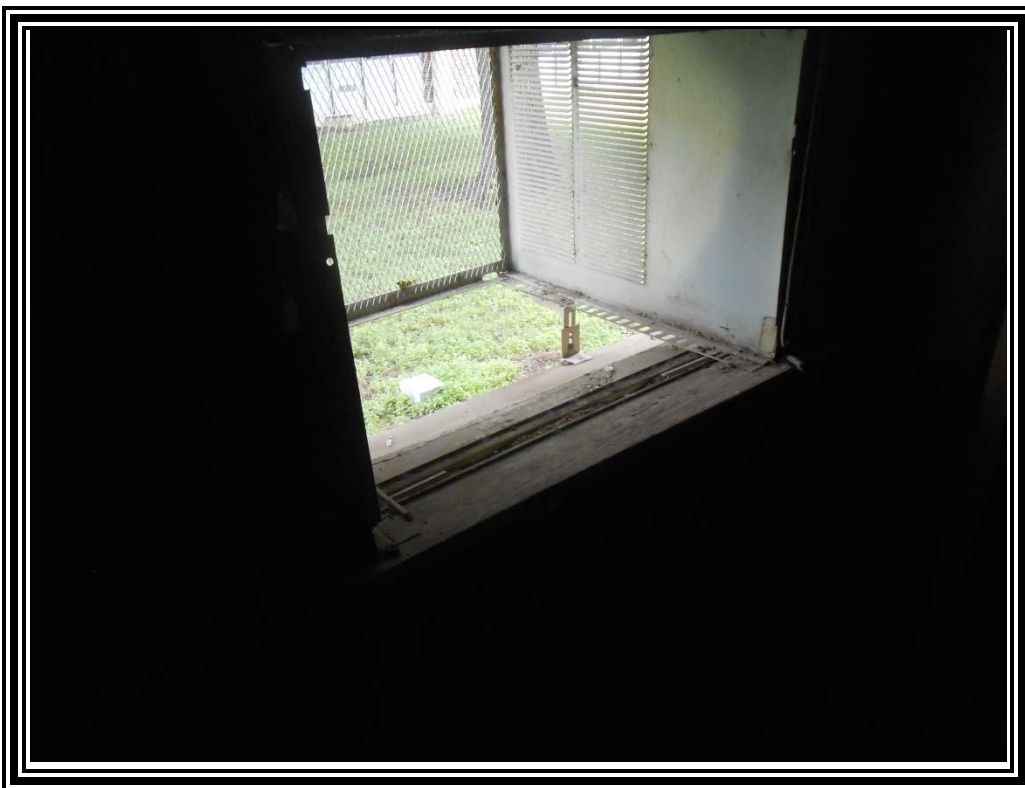
6. View of lead-containing paint on window frame on the exterior of an east side classroom of Margil Hall.
