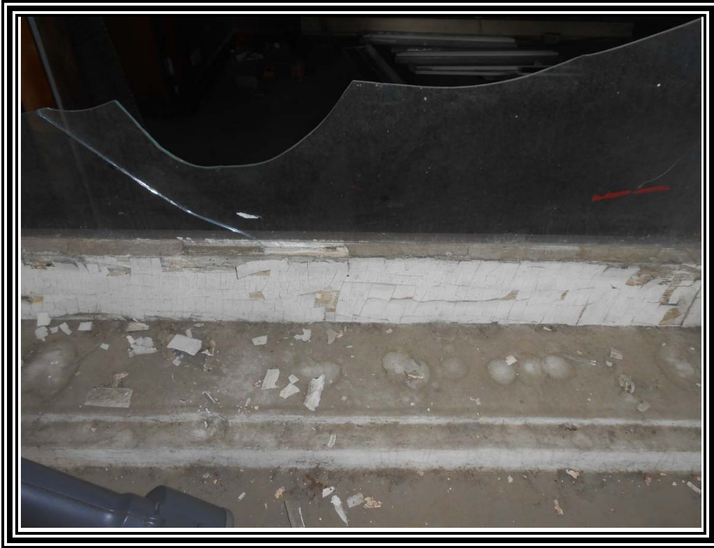
5. View of lead-containing paint on window frame and window sill near the entrance of Margil Hall.
